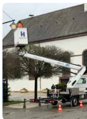
Installation de l'éclairage LED
